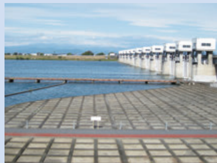
Tone Oozeki barrage for irrigation and municipal water supply
