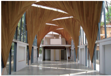
Yayoi Auditorium Annex in the campus of the University of Tokyo using HP shells structure with wood-based materials
